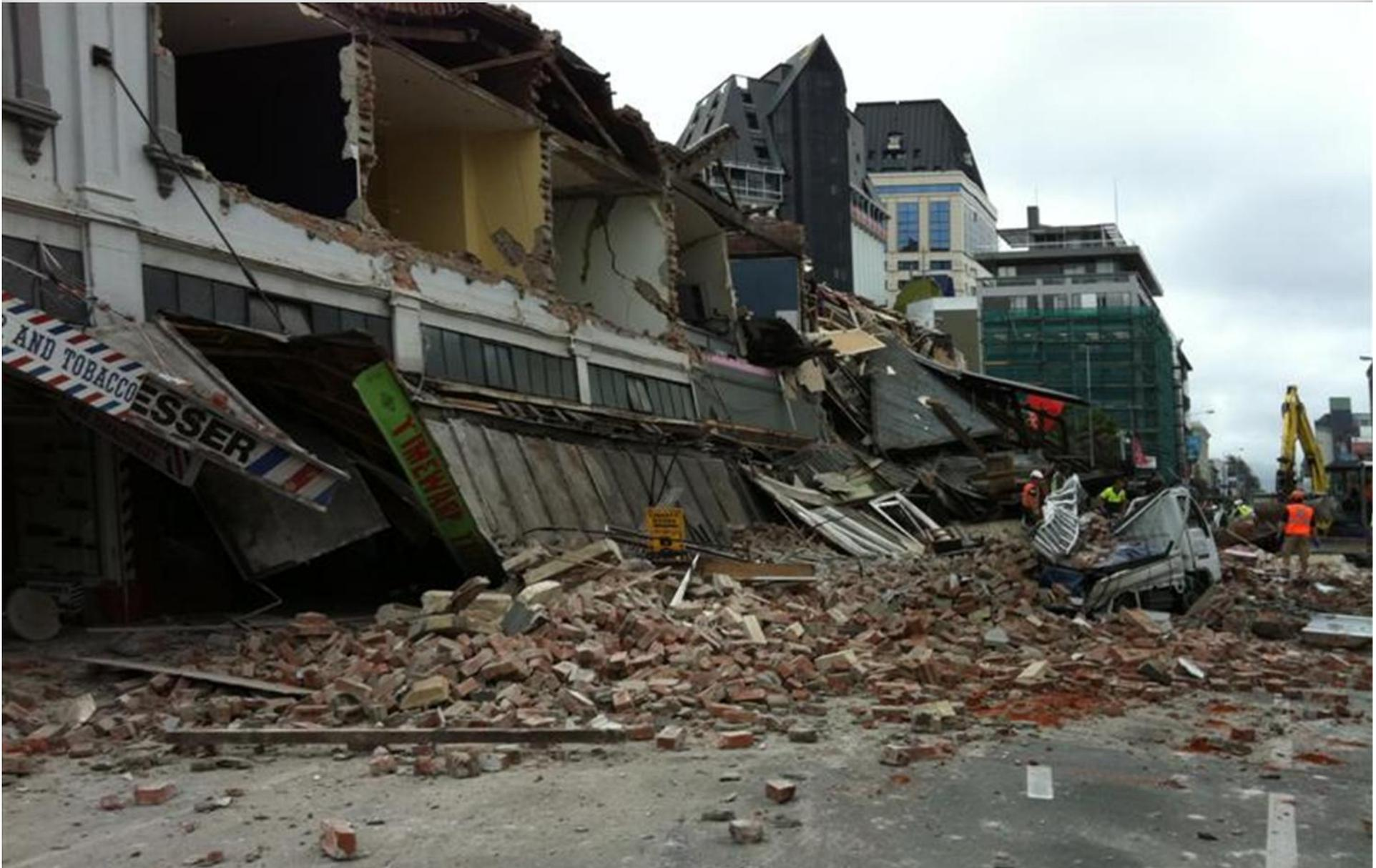
Out-of-plane wall bending failures in Unreinforced Masonry (URM) buildings in Christchurch (42 fatalities)
