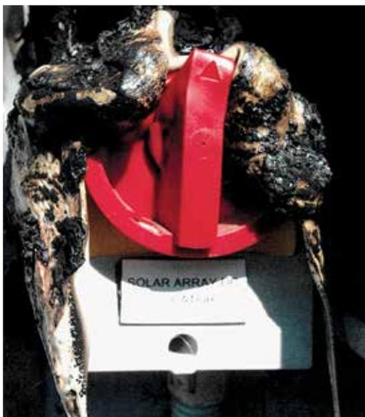
Electrical faults can cause a fire in solar panel arrays, but these are usually sparked by faults in the isolation switch or inverters, rather than the panels themselves.
